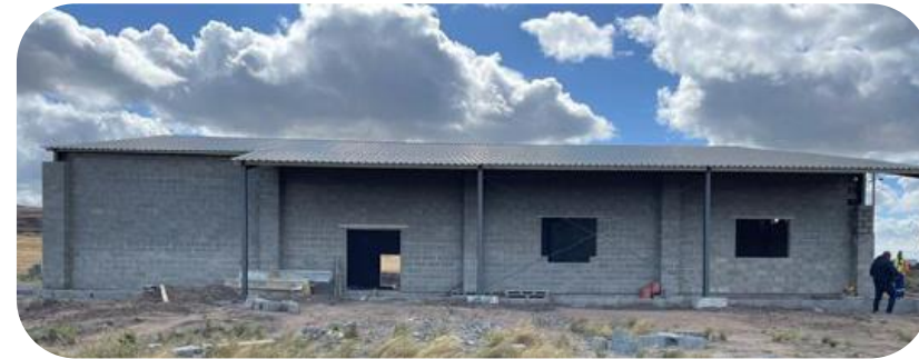
Pondoland Community Centre construction
